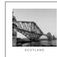
126816 Forth Rail Bridge
